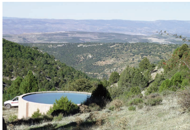
Photo 13: Fire fighting equipments in the Natural Park of Puebla de San Miguel (Valencia Region).
